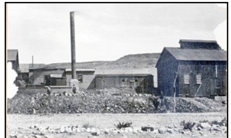
Smelter site in Hillsboro ~1900.
