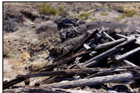
National Defense Mine Complex, east of Hillsboro.
